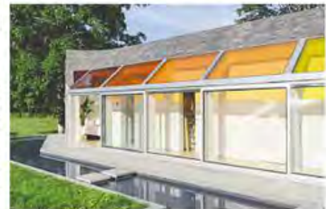
The reflecting pool/cistern collects rain run-off for garden irrigation.
