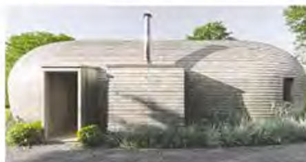
Rounded buildings use up to 20 per cent less material than rectangular structures, make breezes move more efficiently and dissipate sound waves. CARLON HACKWITZ
