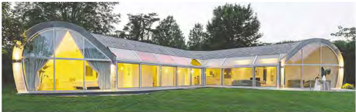
Because it relies on timber rather than steel for its structure, carbon emissions are reduced for this home in Long Island, N.Y.
